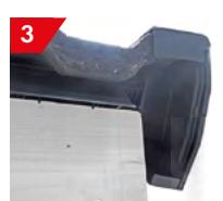
Fit the first verge section ensuring that it is located onto the eaves closer.
