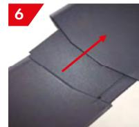
As each successive verge tile is laid, slide on a Uni-Click Dry Verge Unit up to the bottom of the tile, engaging with the Unit below, screw fix into batten ends.
