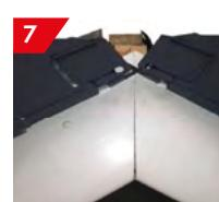
Insert a Ridge Closure into the last unit, interlocking the combs of each Uni-Click Dry Verge Unit at the apex.
