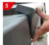
Clip the bottom of the verge unit in place first, then lift the top of the verge unit over and clip in to place. As illustrated in stages 5, 5a and 5b.
