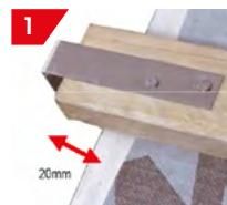
We recommend that the batten is extended 30mm over the barge board or brickwork and 40mm x 3.5mm stainless steel screws (supplied by others) are used to fix the verge units. Prior to fixing the batten, ends must be in good condition with no signs of decay or splitting.
